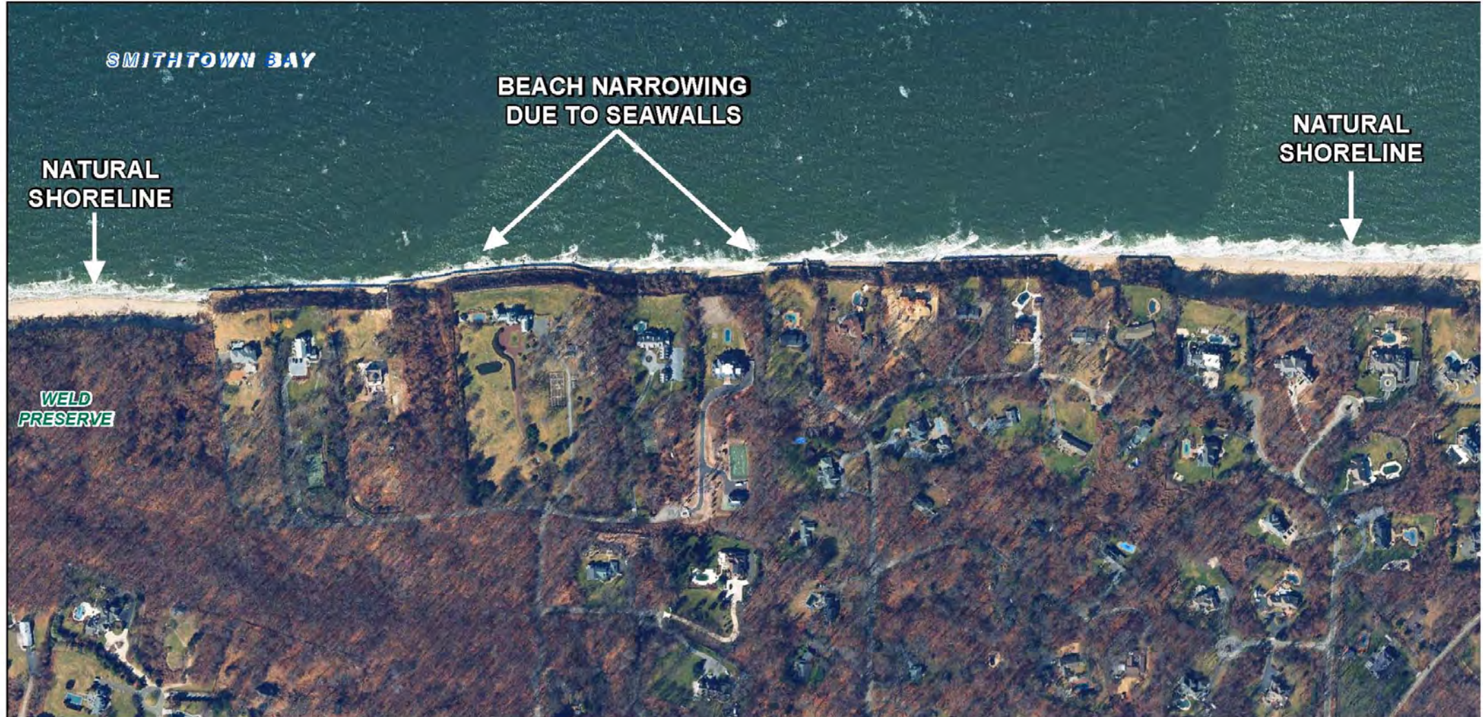
Figure 15. Beach Narrowing in Front of Bulkheads
